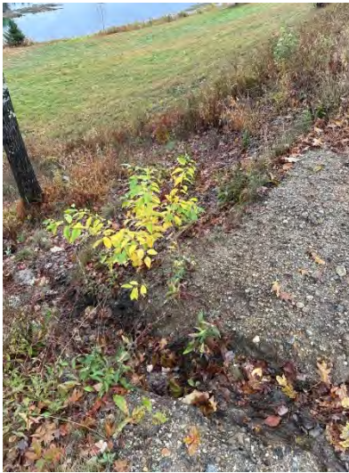
Deep erosion gully that flows into a grassed area along the shoreline of Little Crowcroft Pond with minimal vegetation between the two.
